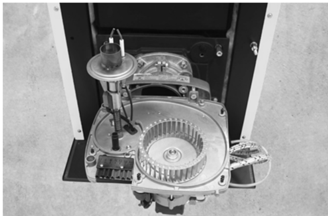
Abb. 36: Brenner in Serviceposition
