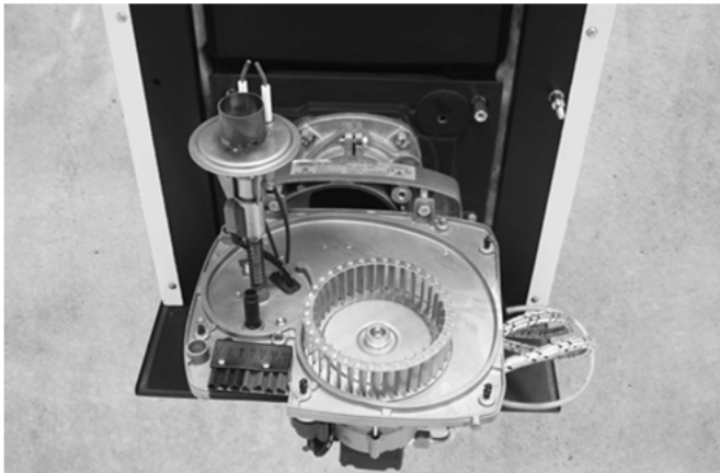
Abb. 36: Brenner in Serviceposition
