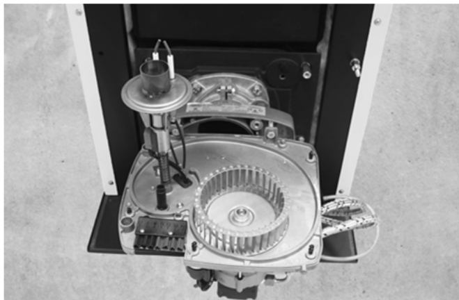
Abb. 36: Brenner in Serviceposition
